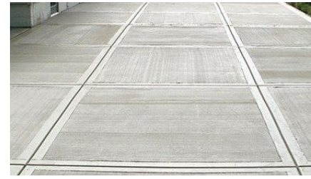
In-situ concrete panels for footpath
