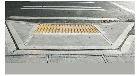
Ramp with drop kerbs and tactile paving for universal accessibility
