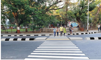
Refuge island for pedestrian crossing
