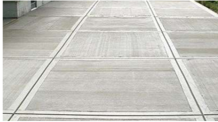
In-situ concrete panels for footpath
